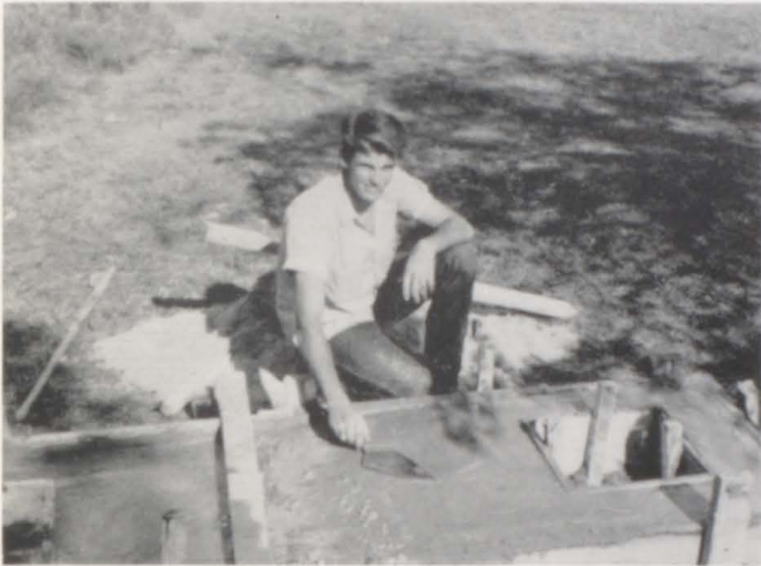
Wayne lays the foundation for the FFA welcome monument.
